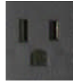
Output receptacles LS 1 - 1 - L5-30R LS 2 - 3 - NEMA 5-15R LS 3 - 3 - NEMA 5-15R
